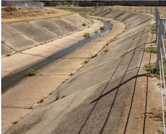
Concretised Stretch of Stony Creek
